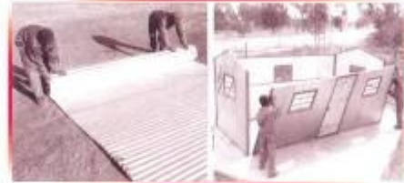
The roof is rolled on like a roll-up garage door
